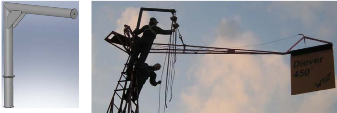
Fig. 4.3: Jib with two chain hoists in series for (rapidly!) hoisting the tail (photo 2005)
