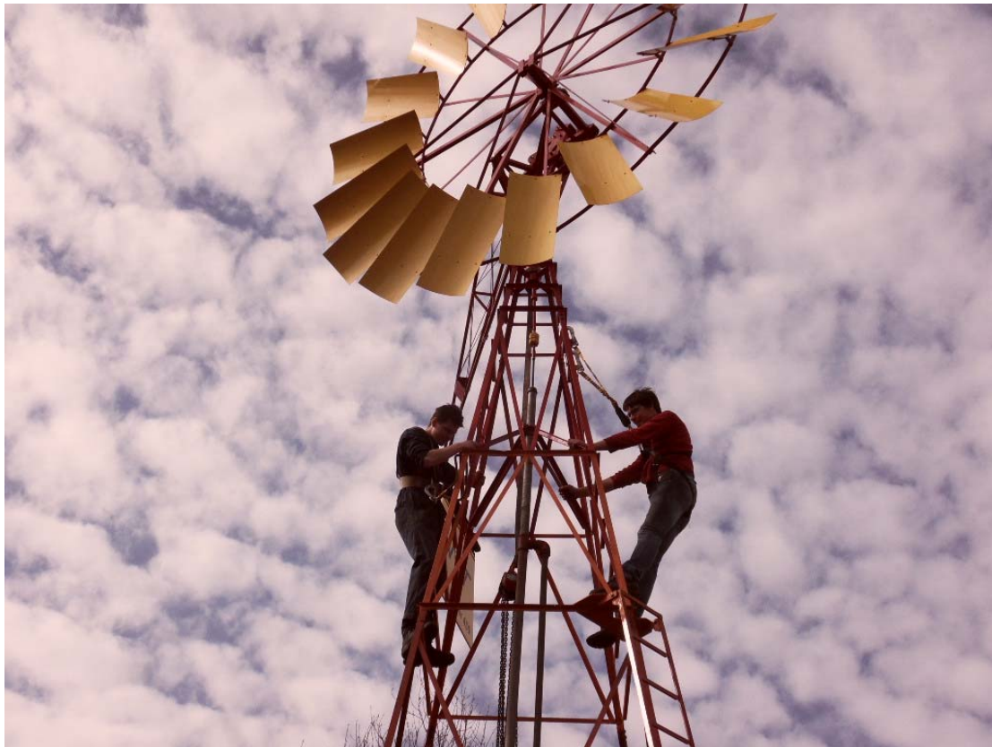
Fig. 0.1: installing of pump (photo 2016)
