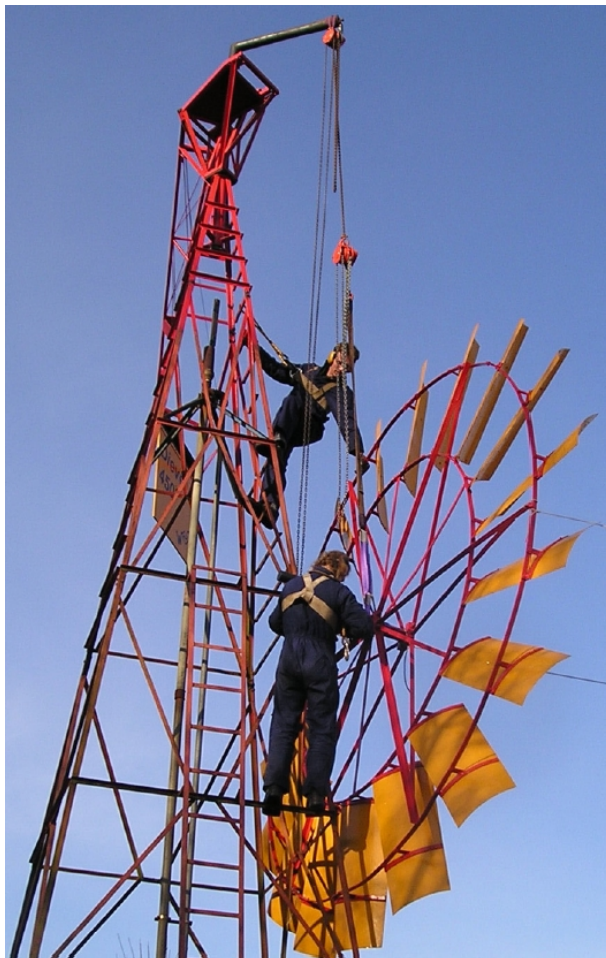
Fig. 0.2: hoisting of rotor (photo 2005)
